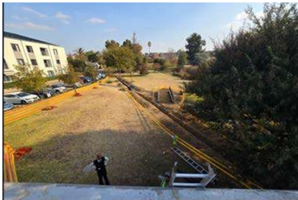
Trenching from LSC to the gate (Showing the new bridge).
