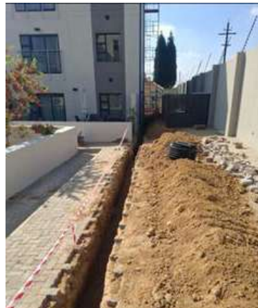
Washing lines excavation
