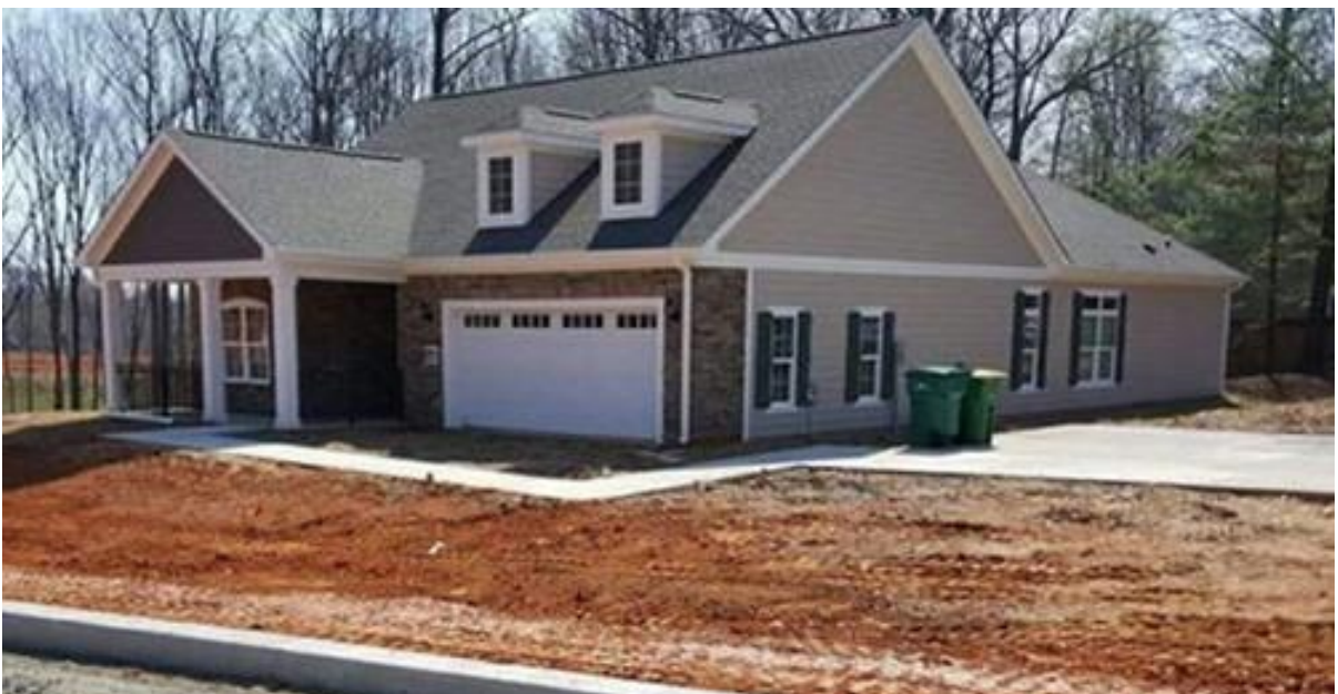
Side entry garage
